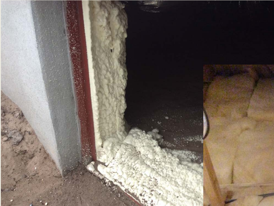
Closed Crawl Space with Spray Foam Walls
